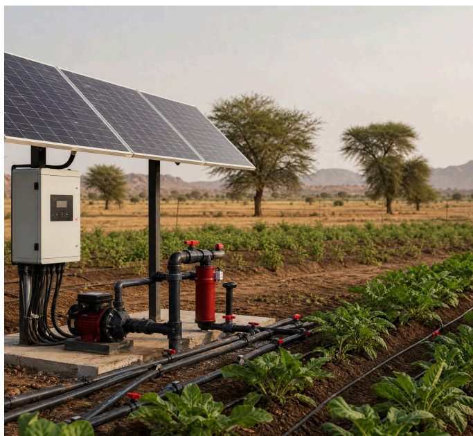
Solar-supported irrigation, filtration, pumping and drip delivery represented as an integrated field system.
